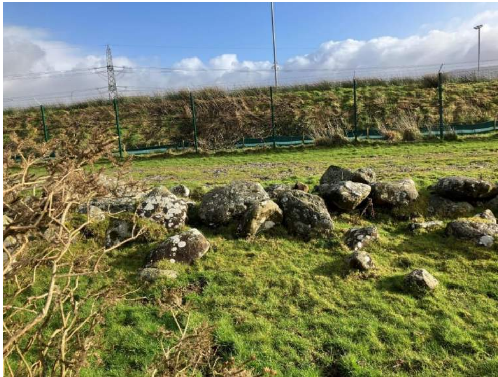
Photograph 8: North facing shot of substation and stone wall at edge of site.
