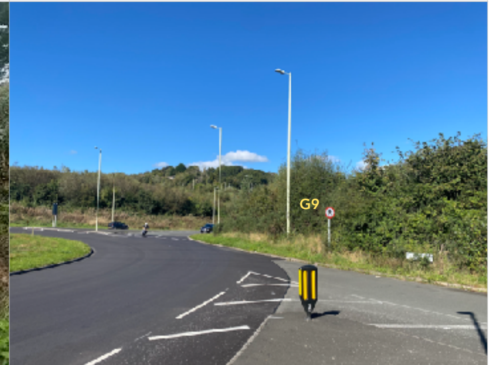
IMAGE 6: G9 facing north from Pound Farm Lane onto the A473.
