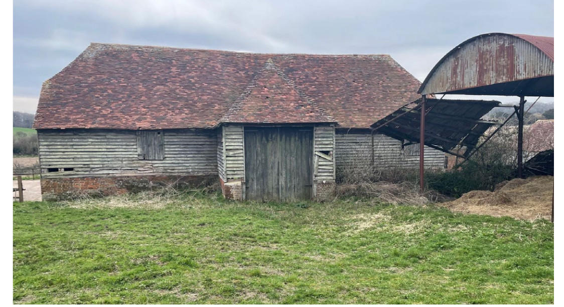
Existing Tithe Barn & Dilapidated Dutch Barn
