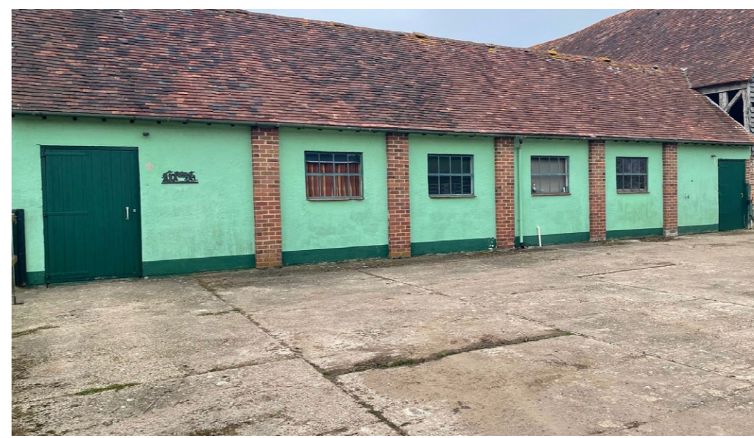
View Of Existing East Elevation
