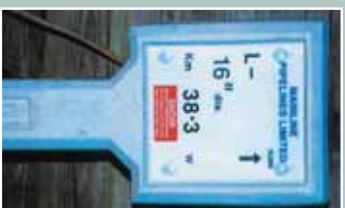
Mainline marker post
