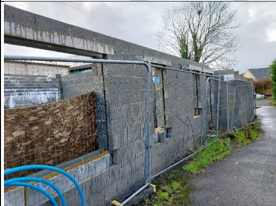
Figure 18 - Current state of building E
