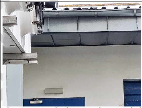
Figure 7 - Ventilation covering of building A
