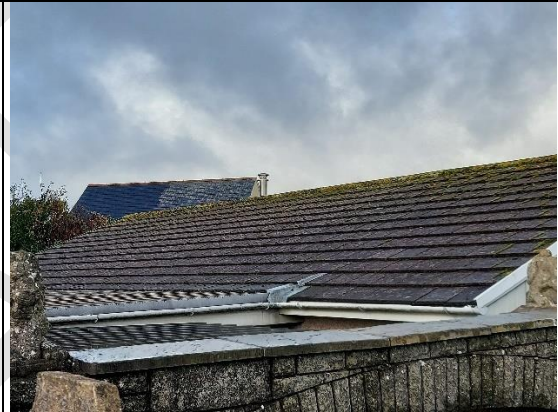
Figure 11 - West elevation roof of building B
