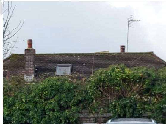
Figure 13 - Eastern elevation roof of building C
