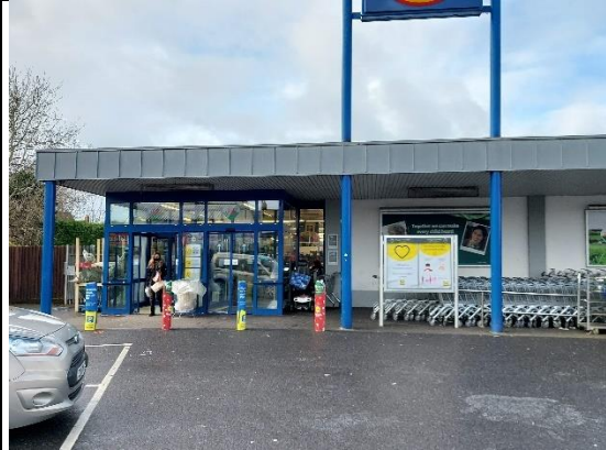
Figure 4 - Eastern entrance to building A
