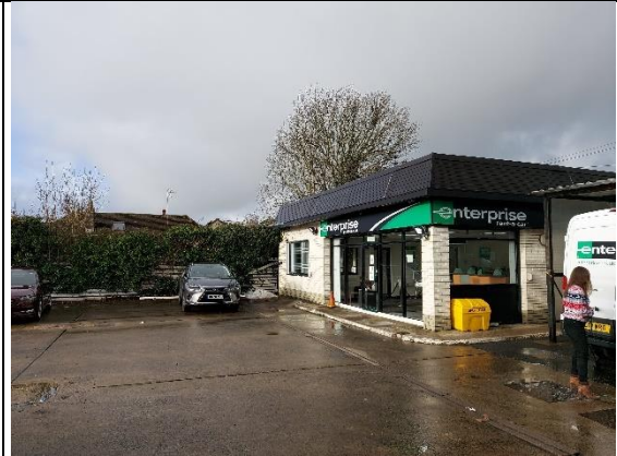
Figure 15 - South-east corner of building D
