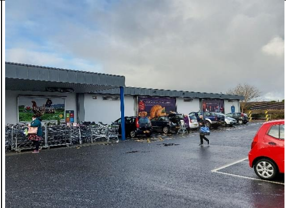
Figure 5 - Eastern elevation of building A
