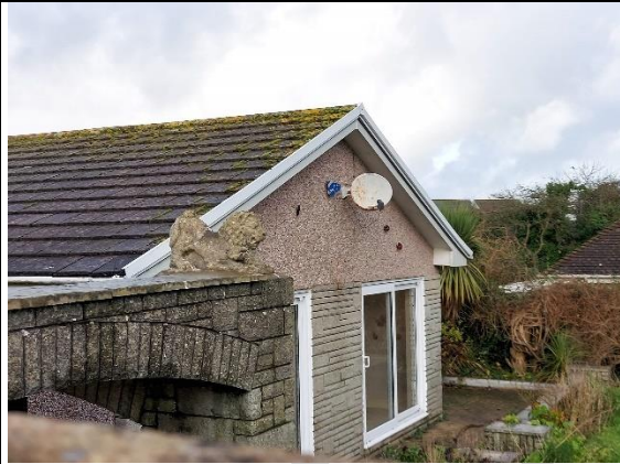
Figure 10 - Southern gable end of building B
