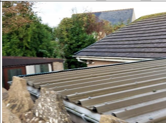
Figure 12 - Roof of the extension and outbuilding at building B
