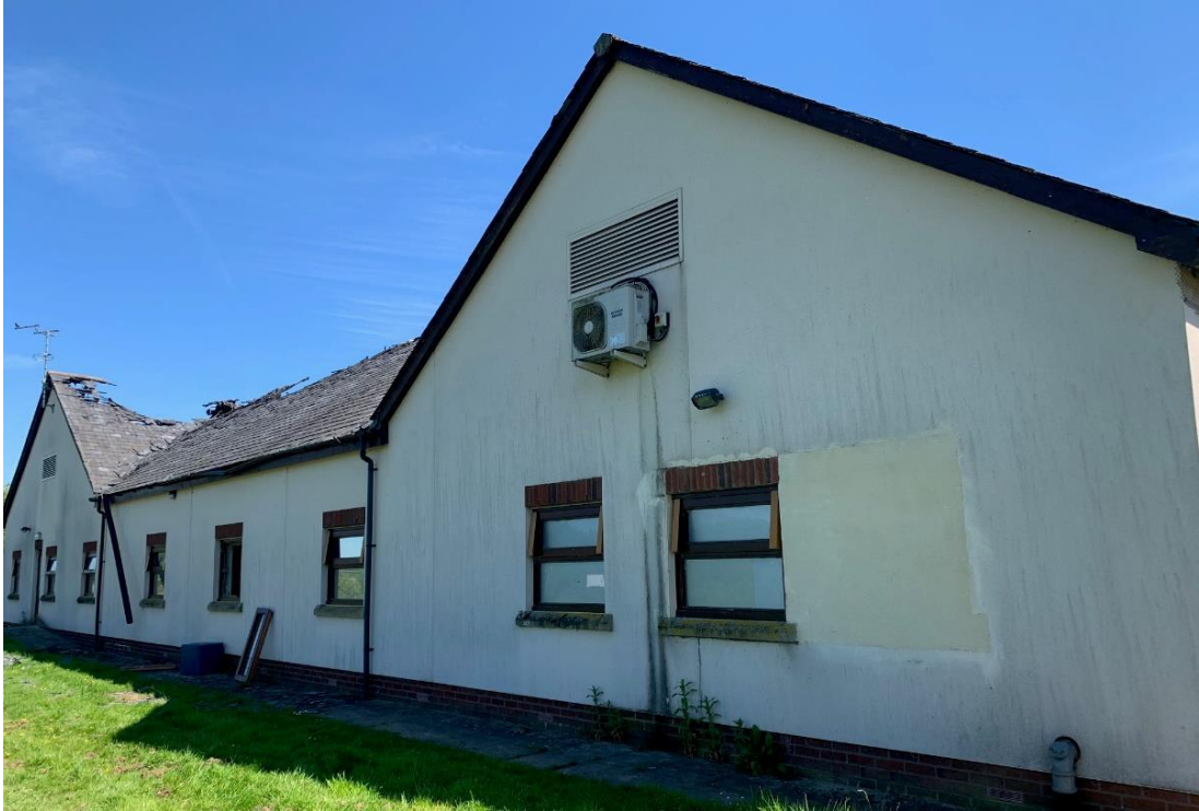
Figure 3: Former Treowen Building – NE Elevation
